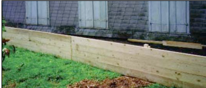
Figure 18. Emergency plate system (VKF / BWG, 2004b)
