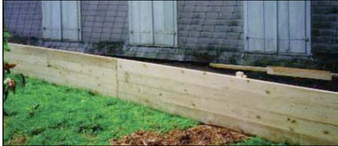
Figure 18. Emergency plate system (VKF / BWG, 2004b)
