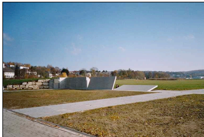
Figure 3. Completely preinstalled stationary flap system in Sinsheim near Heilbronn, Germany (KWS, 2010)
