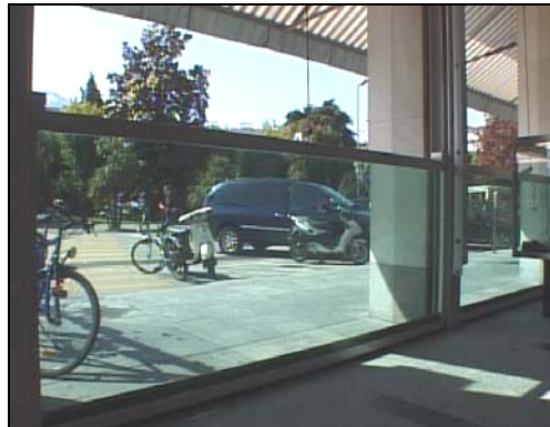
Figure 5. Lowerable glass segment system in protection position in a parking deck in Locarno, Switzerland (KWS, 2010)
